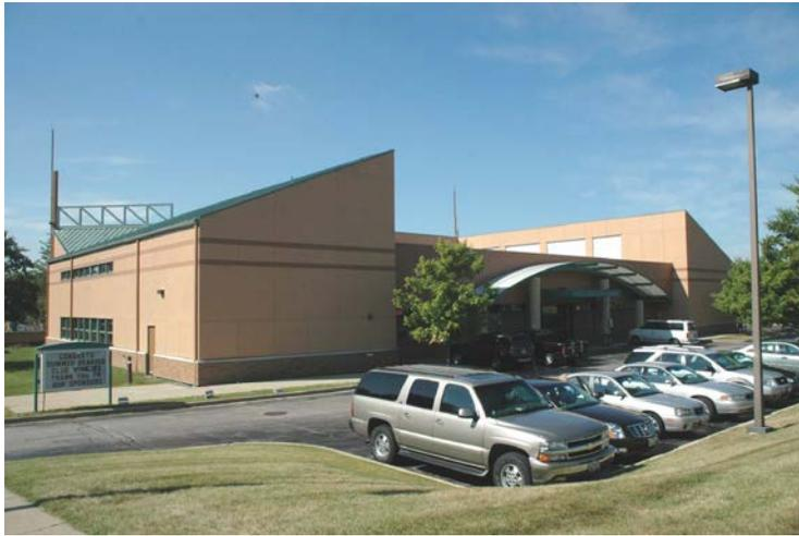
The Itasca Community Library originally consisted of a 1-story steel-framed structure with a low-slope roof and masonry exterior walls. In 1996, the library was renovated and expanded. The addition consisted of a 2-story steel-framed structure along the east, south, and west sides of the original building. A comprehensive facade rehabilitation project was completed in 2009 to address significant water leakage issues associated with the exterior walls and roof of the addition.
