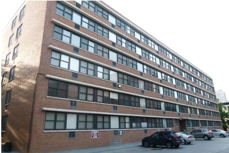
Originally constructed in the 1950s, the 7-story residential building at 2300 North Commonwealth Avenue consists of a reinforced concrete structure. Exterior walls have generally been constructed using multi-wythe brick masonry. The roof of the building consists of a low-slope modified bitumen roofing system with an outdoor deck area.
