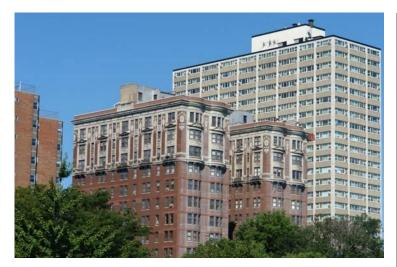
Located at 5000 North Marine Drive, The Aquitania Building is a 15-story concrete framed structure built in the mid-1920s. The exterior facade of the building is clad in architectural terra cotta, brick, and limestone masonry. The Aquitania Building is designated as an Illinois Historic Landmark.
