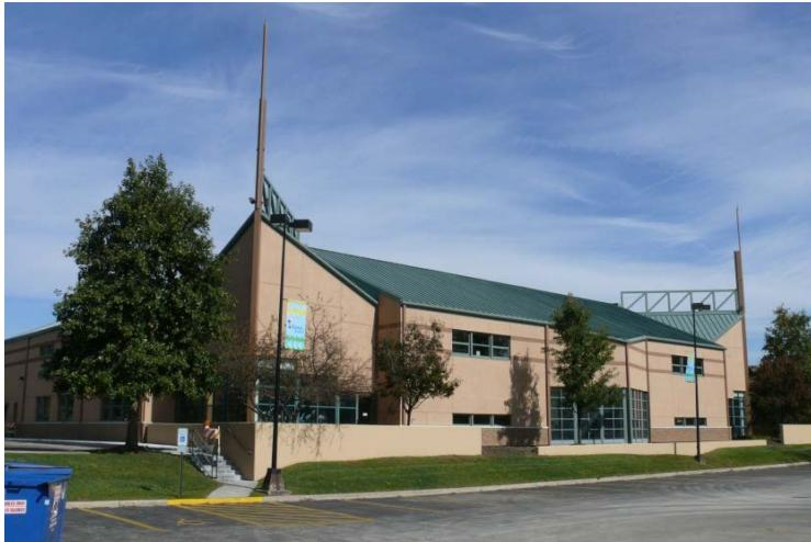
The original Itasca Community Library building consisted of a 1-story steel-framed structure with a low-slope roof and masonry exterior walls. In 1996, the library was renovated and expanded. The addition consisted of a 2-story steel-framed structure along the east, south, and west sides of the original building. The addition exterior walls were clad with a direct-applied exterior finish system (DEFS), and a steep-slope architectural standing seam metal roofing system.
