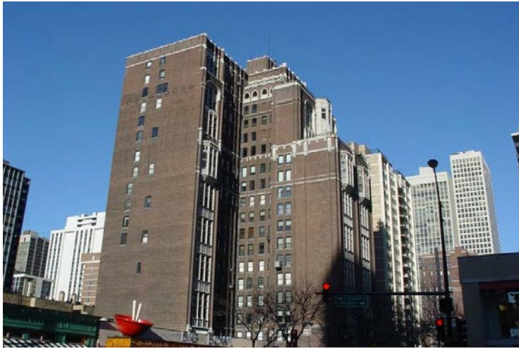
The 20 East Cedar Building is a 19-story gothic high rise completed in 1925. The center of the building steps back at the south elevation to form terraces at the 14<sup>th</sup> and 18<sup>th</sup> floors. The building is concrete framed and clad in brick and architectural terra cotta. The south elevation also includes four 2-story terra cotta clad Oriol windows, a projecting terra cotta clad spiral stairway enclosure, and 7 large finials at the 14<sup>th</sup> floor terrace.
