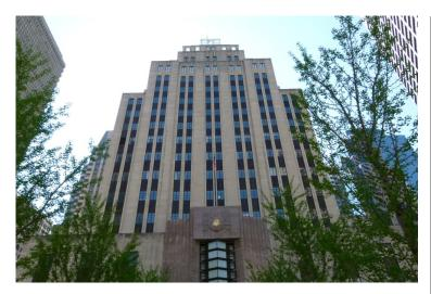
The 185 Franklin Street Building is a 22-story steel-framed structure originally built in 1947. A 14-story addition was constructed in 1970. The exterior walls of the original building and the addition consist of solid masonry with a limestone exterior wythe.
