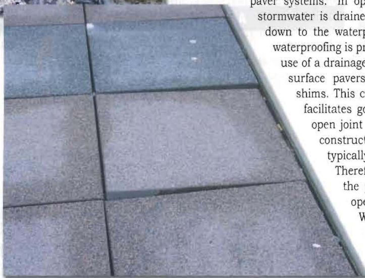
Shifting and rocking of pedestal supported pavers.
