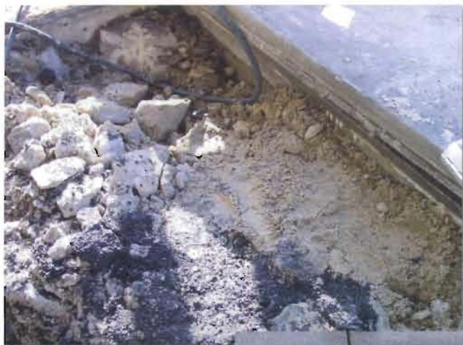
Extensive deterioration of a plaza deck mortar setting bed in a closed joint system. The plaza is located in a cold region.
