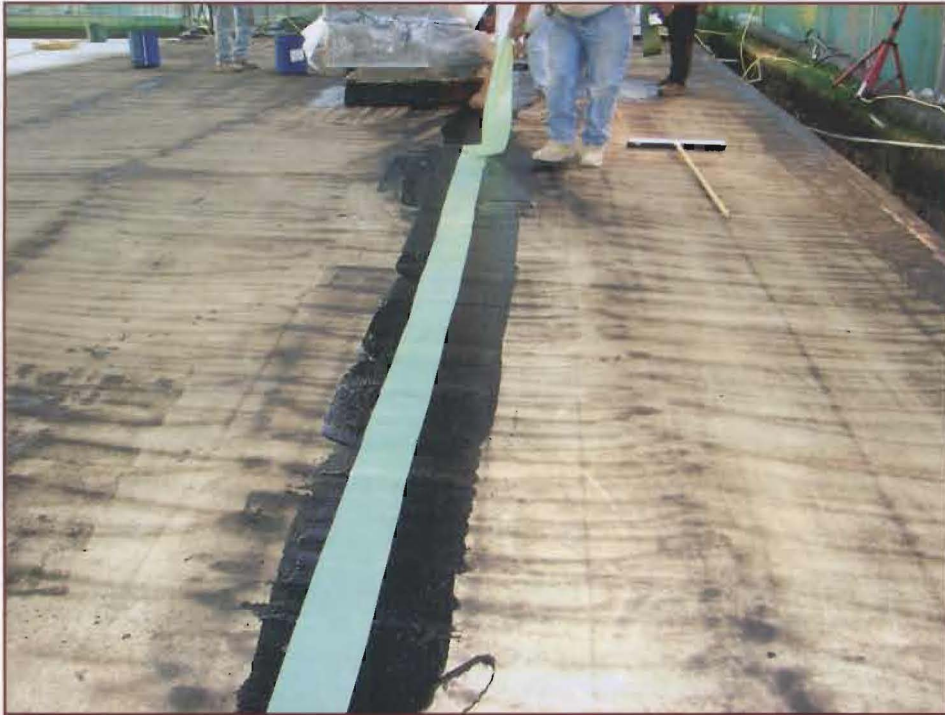
Photo 8: Each manufacturer's requirement for substrate crack treatment varies. Designers should take the most conservative approach in addressing substrate cracks to avoid future problems.
