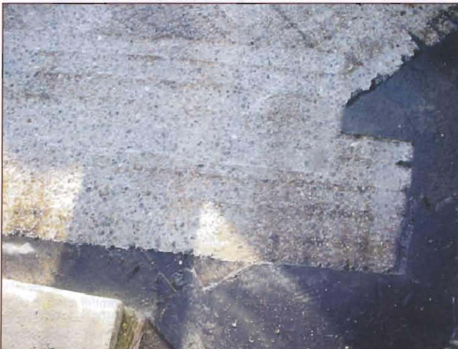
Photo 6: Scarifying is a good method for removal of an existing adhered waterproofing membrane. However, care should be taken to avoid over-roughening of the substrate.
