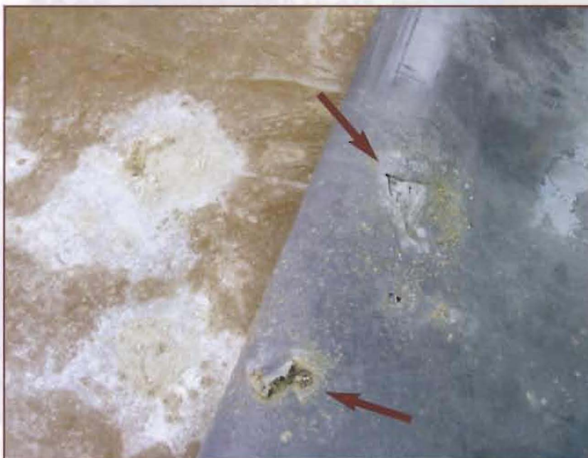
Photo 5: Inadequate surface preparation can lead to problems. Small pieces of gravel left on the surface can lead to punctures in the membrane.
