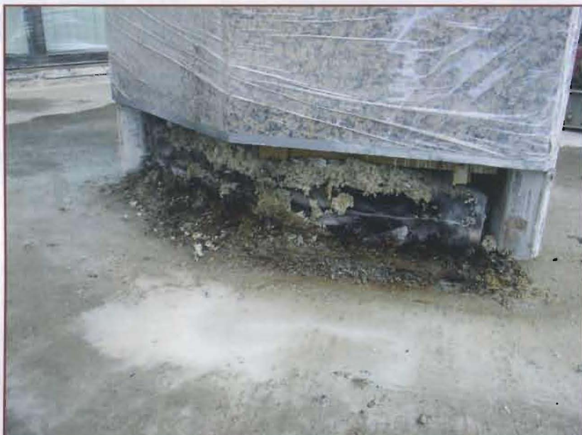
Photo 3: In many cases, original waterproofing system base flashings are installed prior to many exterior components, such as column cladding. In such cases, column claddings and curtain wall bases will have to be modified so that new base flashing can be installed.
