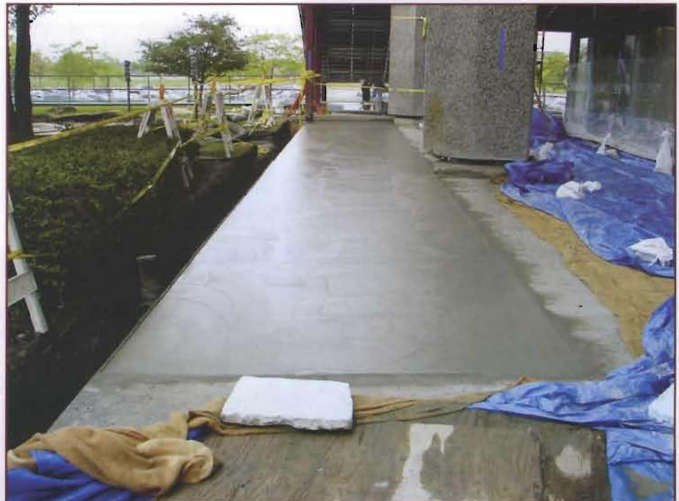
Photo 2: A cementitious tapered topping can be installed in some cases to improve subsurface drainage. Note the previously placed areas to the right are being moist cured with burlap and plastic sheets.
