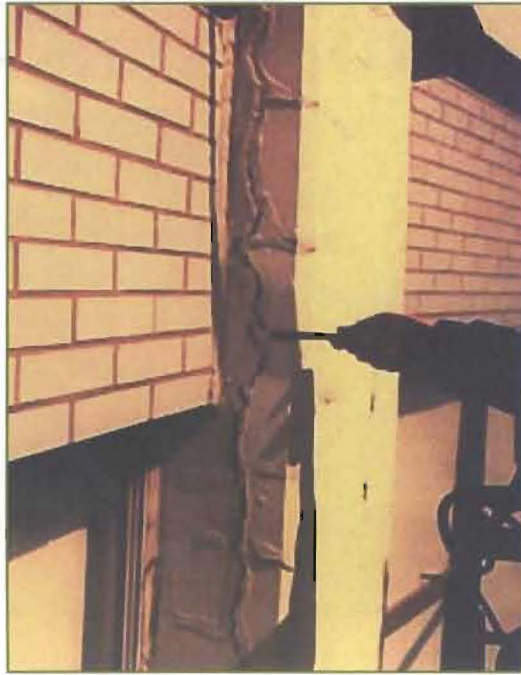
Photo 3 – Indications of extensive reinforcing-steel corrosion on a high-rise building exterior column.
