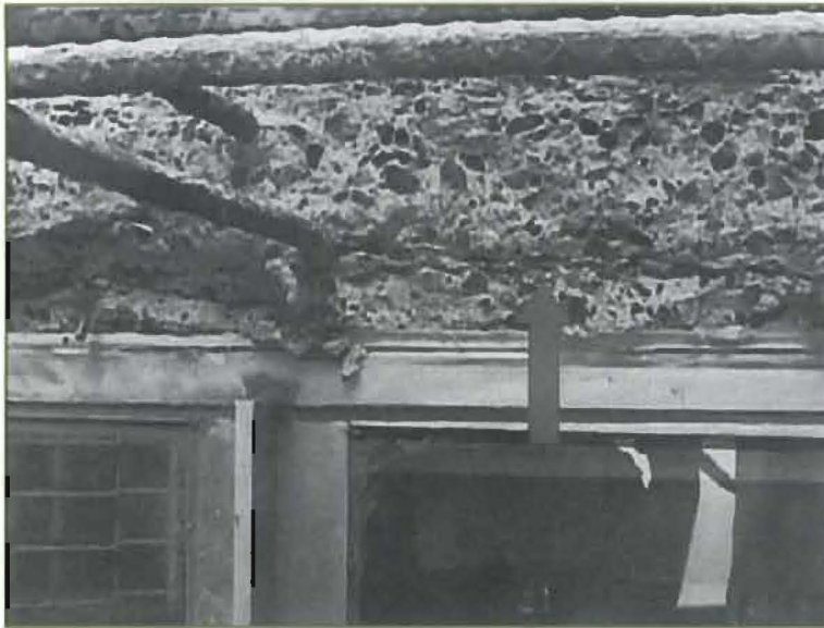
Photo 12 – Corrosion-related delamination that has extended inside the building.
