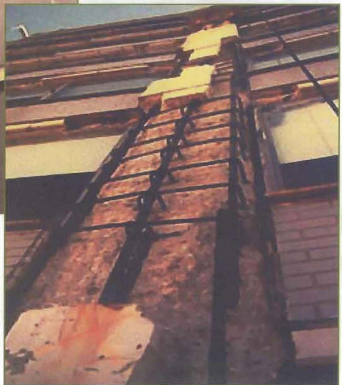
Photo 5 – Same column shown in Photo 3 during repairs.
