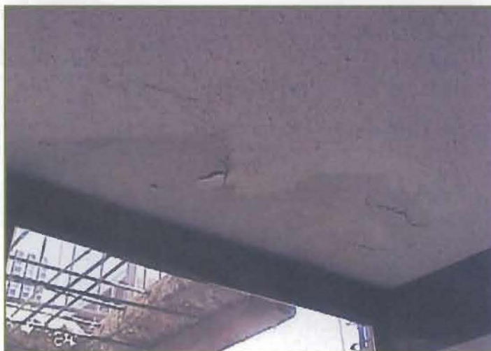
Photo 10 – Early indications of reinforcing steel corrosion inside a building adjacent to an exterior window.
