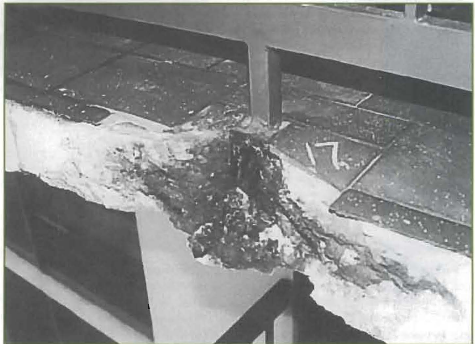
Photo 8 – Typical deterioration of balcony railing pockets.
