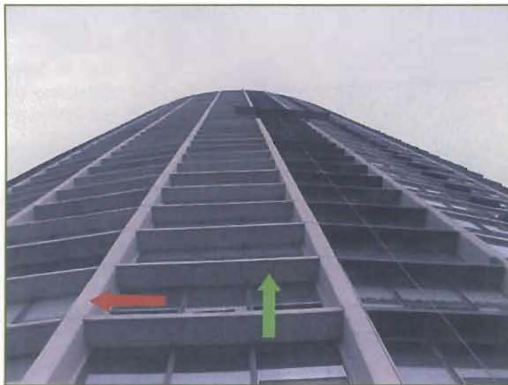
Photo 1 – High-rise building with exposed cast-in-place concrete columns (red arrow) and slab extensions (green arrow).
