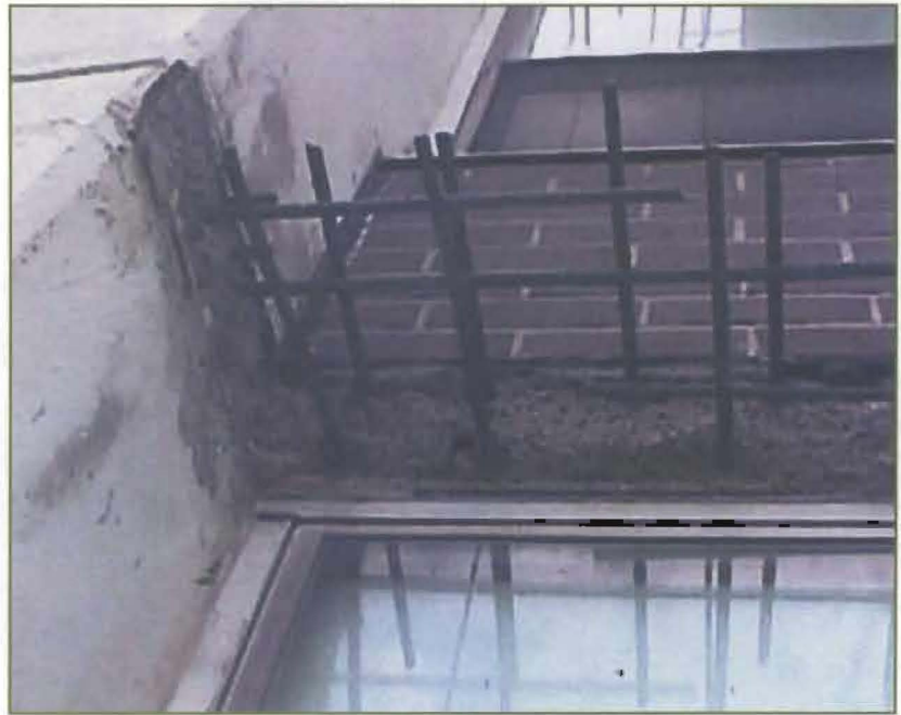
Photo 9 – Removal of slab extensions adjacent to columns during repairs can lead to a significant reduction in shear transfer capacity at the column-slab connection.
