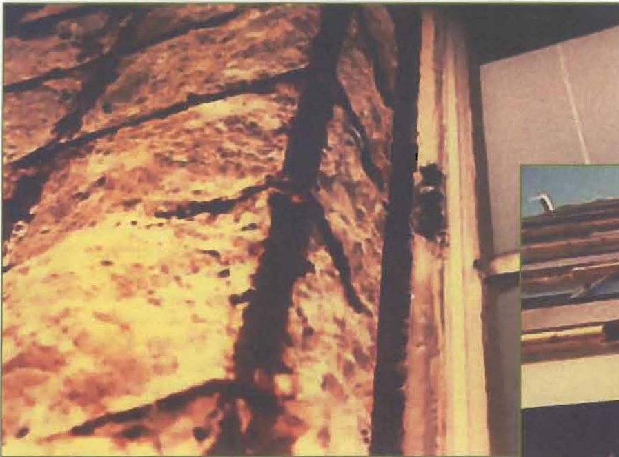
Photo 4 – Same column shown in Photo 3 after removal of the delaminated concrete.
