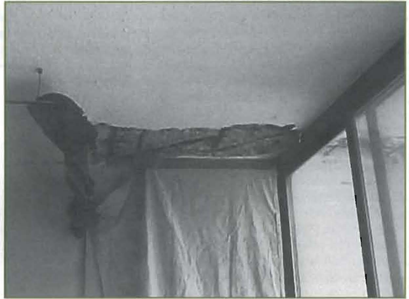
Photo 11 – Corrosion of reinforcing steel that has extended inside a building.
