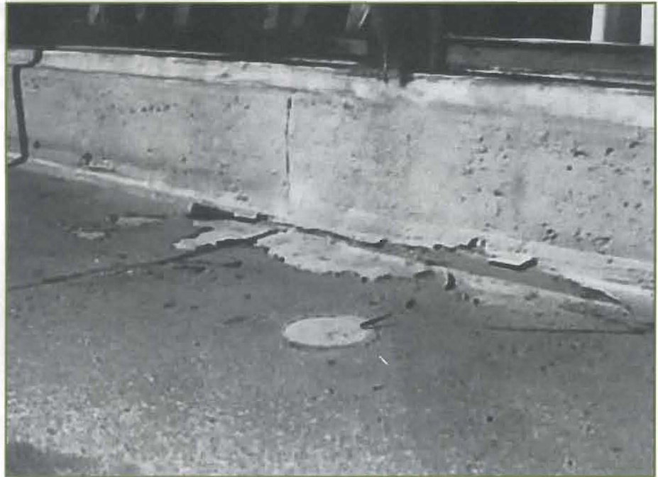
Photo 7 – Failure of protective coating on a slab extension.
