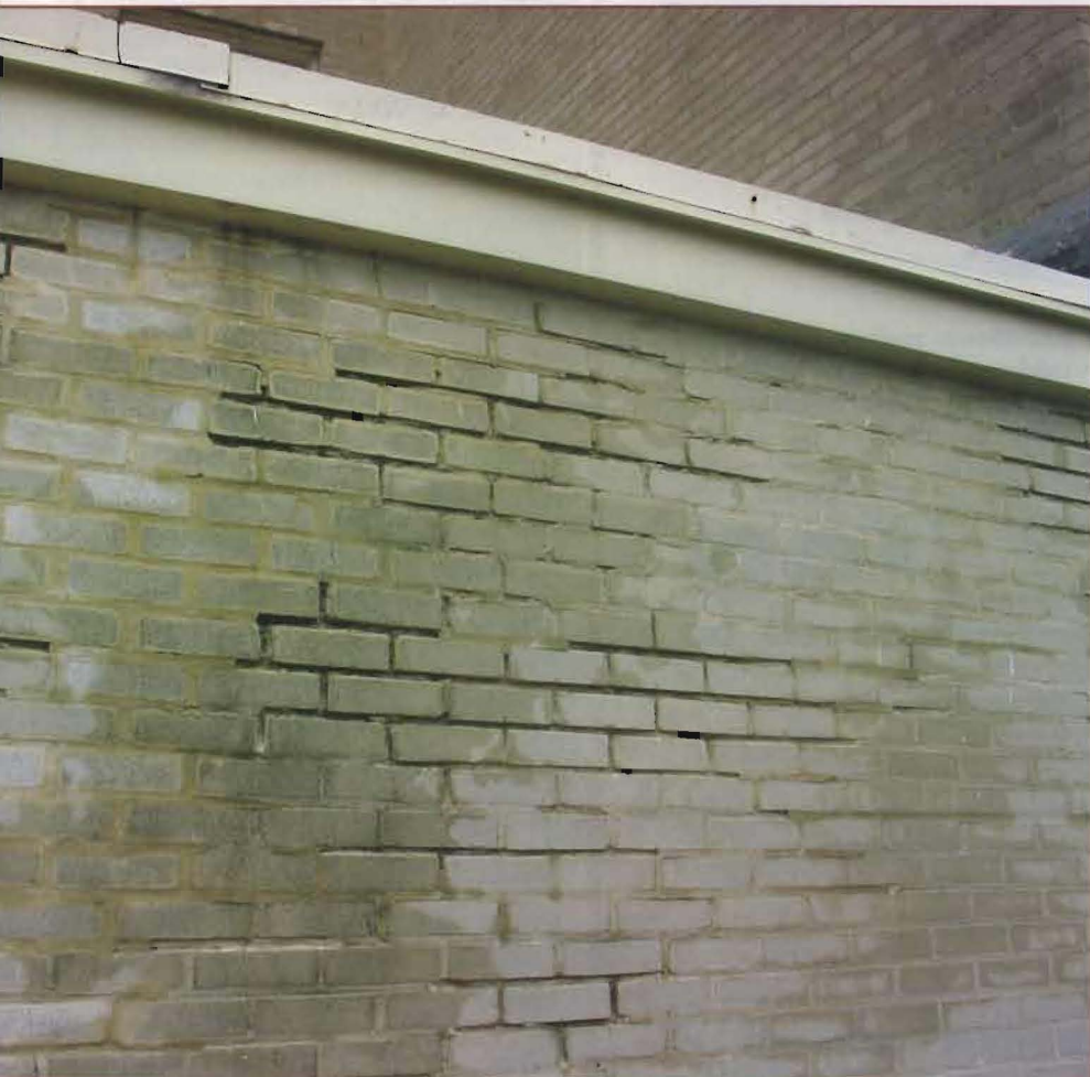
Photo 4: Freeze-thaw deteriorated mortar joints.
