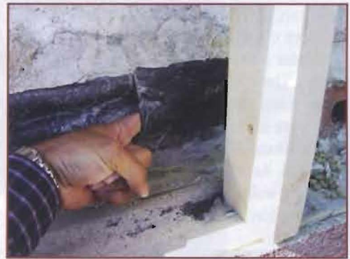
Photo 6: Improperly sealed flashing seam.
