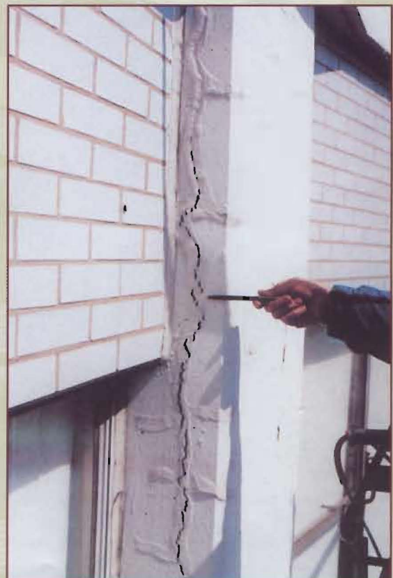
Figure 2 - Cracking associated with extensive corrosion of the vertical reinforcing bars in a concrete column (approximately 20 stories high).
