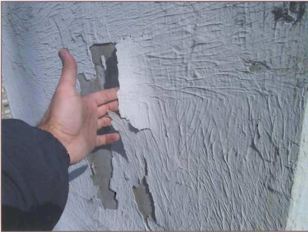
Figure 4 - Coating failure on a concrete shear wall on a high-rise facade.
