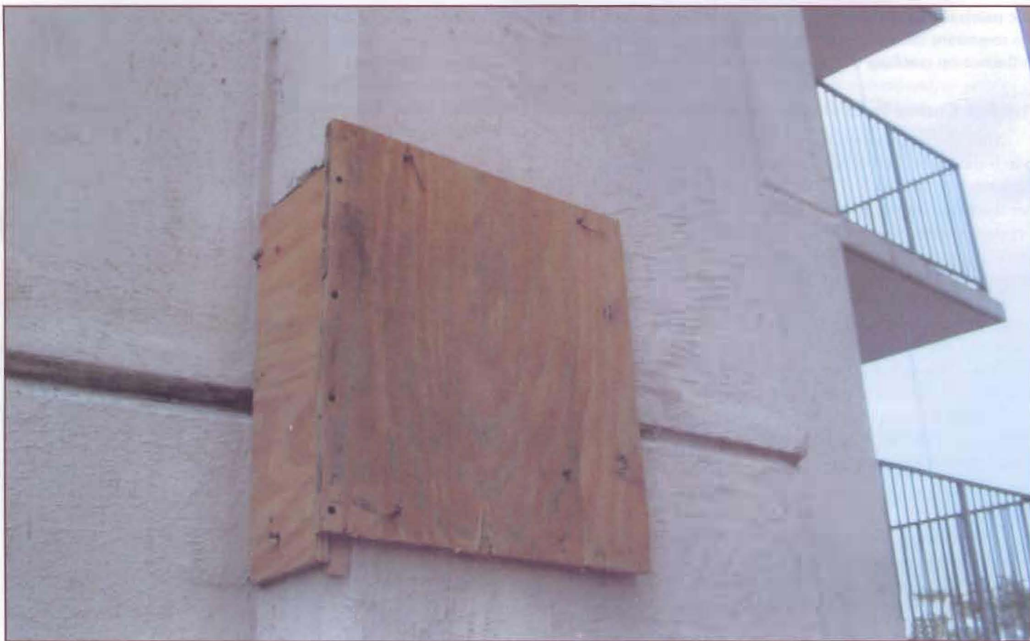
Figure 8 - Forming of a concrete column patch.
