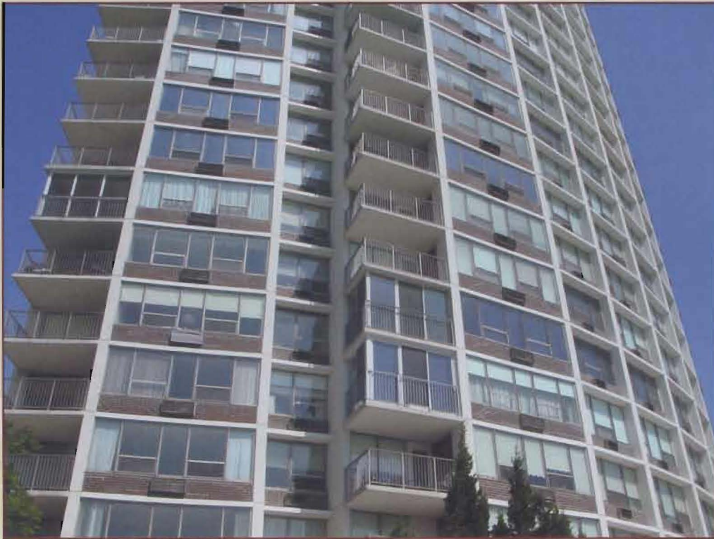
Figure 1 – Typical high-rise building facade with exposed concrete structural elements such as slab edges, columns, and balconies (painted white).
