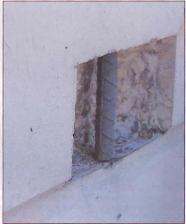
Figure 6 - Small patch area. Note the perimeter saw cut has been dovetailed to lock the patch material in place. Also, the depth of saw cut has been reduced due to shallow concrete cover at the reinforcing steel.
