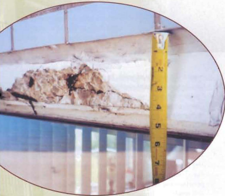
Figure 3 - Concrete spalling at an exposed slab edge due to corrosion of reinforcing steel.
