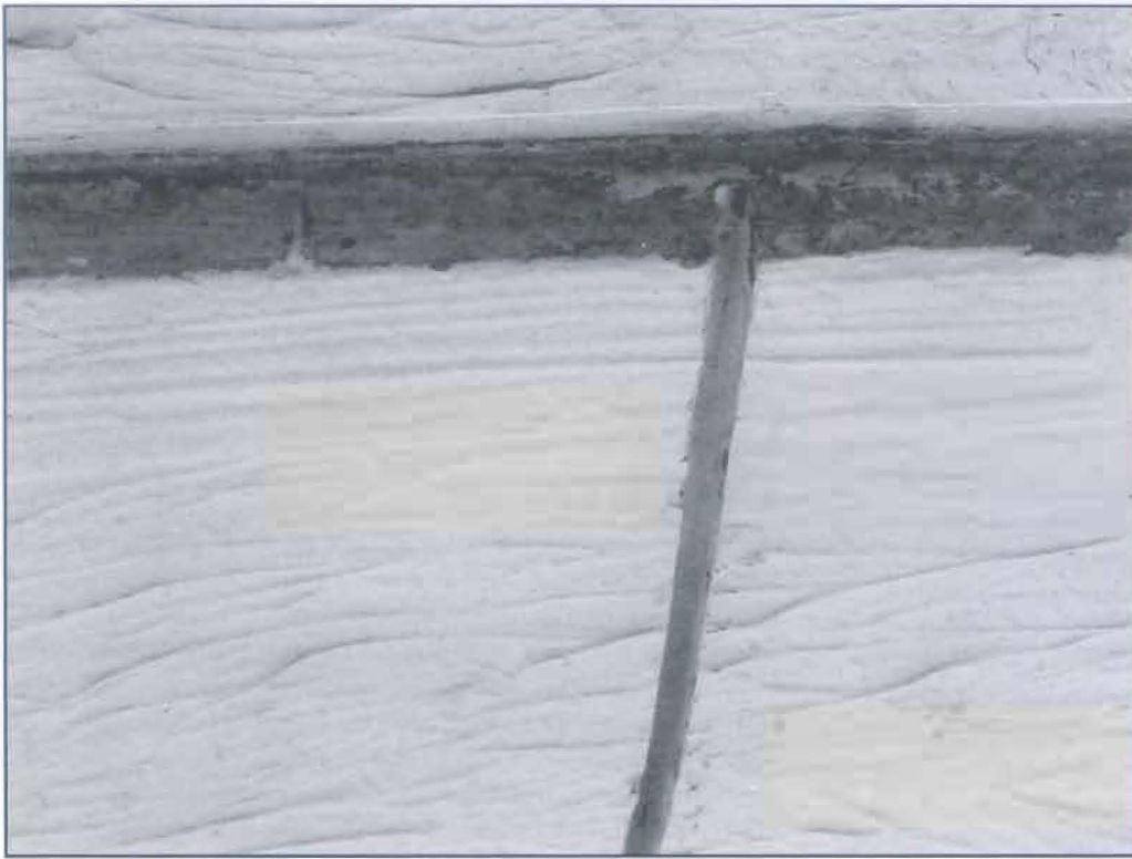
Figure 9 - A routed crack prior to installation of the backer rod and sealant.
