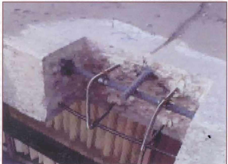
Figure 7 - Stainless steel supplemental reinforcing steel installed at a repair location.
