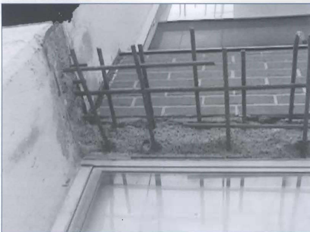
Figure 5 - When removing concrete at slab-column interface, shear transfer at the connection should be considered.
