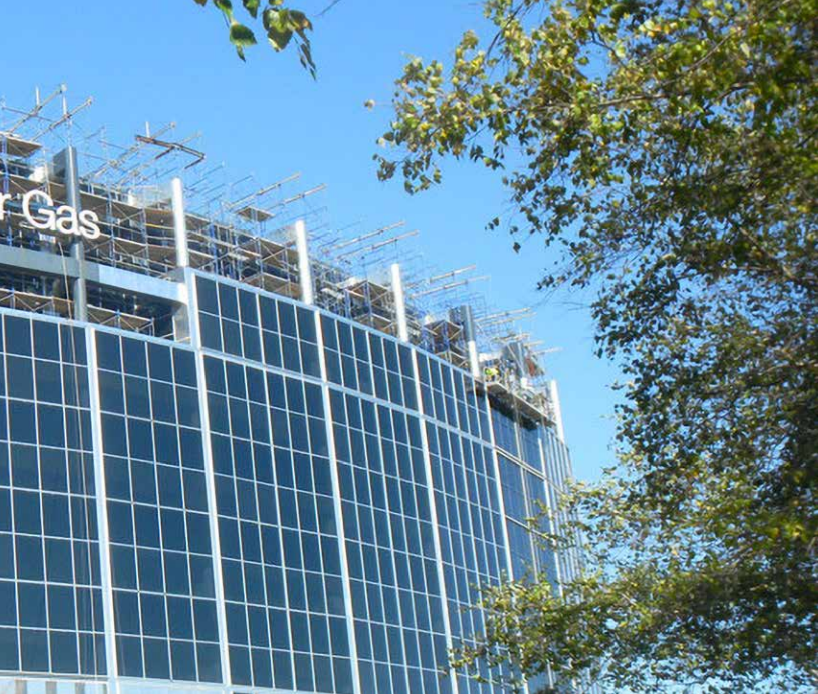
Photo 2: View of the building corner showing barrier-type metal panel cladding at corners (yellow arrow) and buttresses (red arrow). East and west elevations of the building also included HVAC
