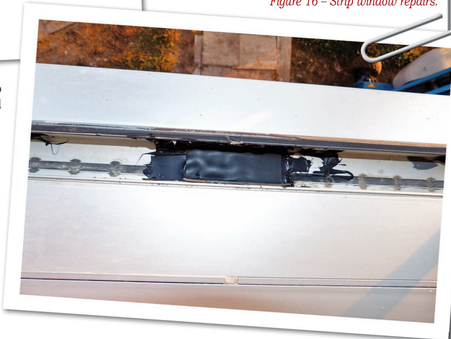
Figure 16 – Strip window repairs.
