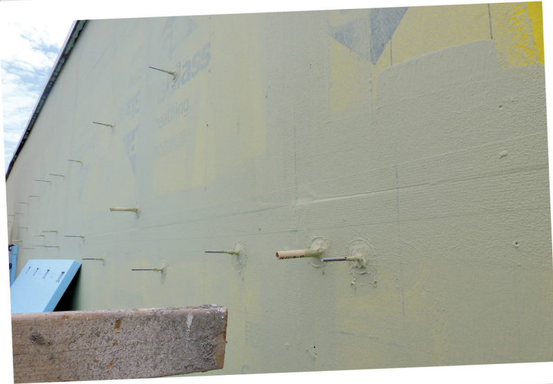
Figure 13 – WRB application around signage support anchors.
