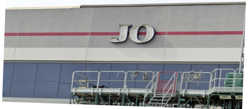
Figure 14 – Reinstallation of signage over finished stucco cladding.
