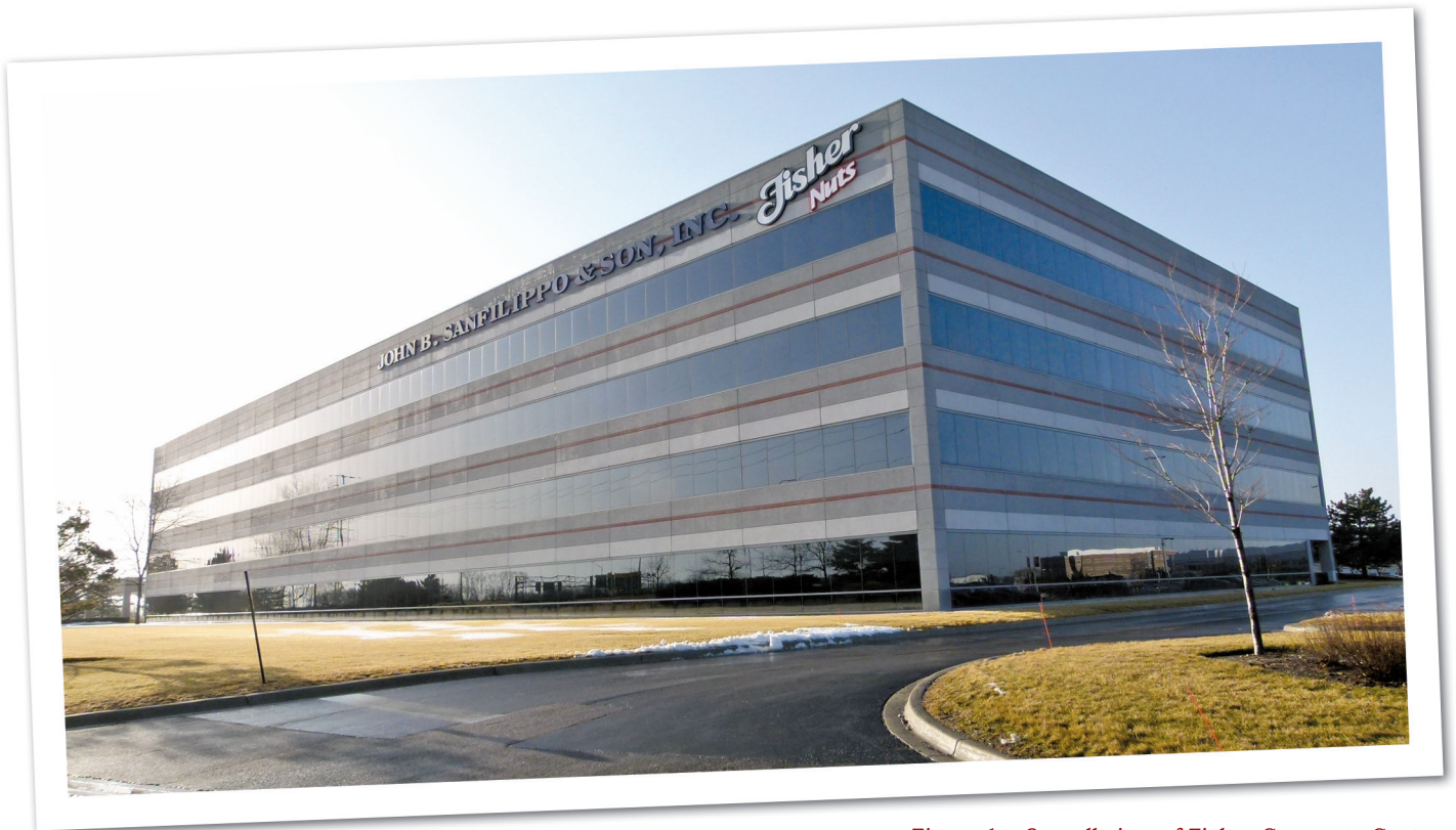
Figure 1 – Overall view of Fisher Corporate Center.
