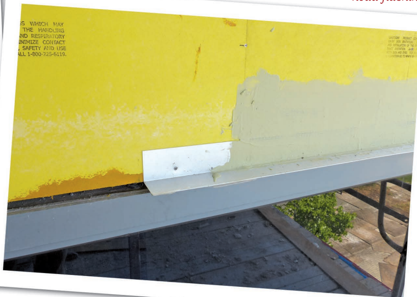
Figure 10 – Window head flashing.
