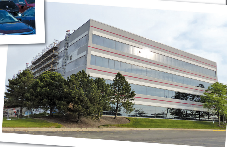
Figure 18 – Completed east elevation.
