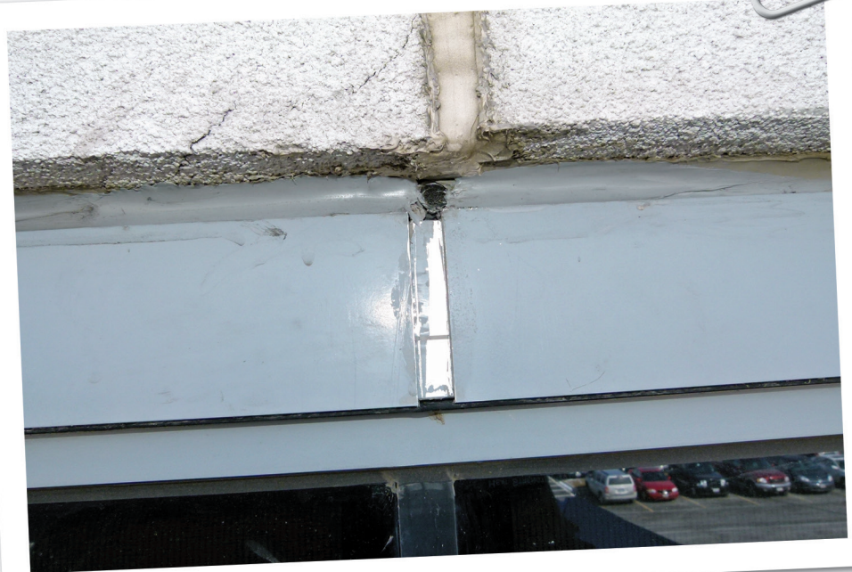
Figure 4 – Splice joint with no cover plate.
