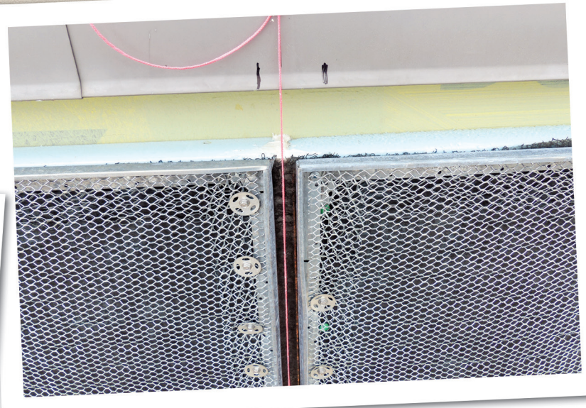
Figure 12 – Metal lath fasteners spanning across insulation and sheathing.
