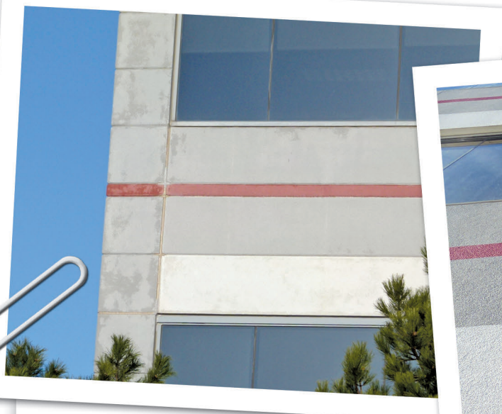
Figure 7 – Original EIFS cladding.
