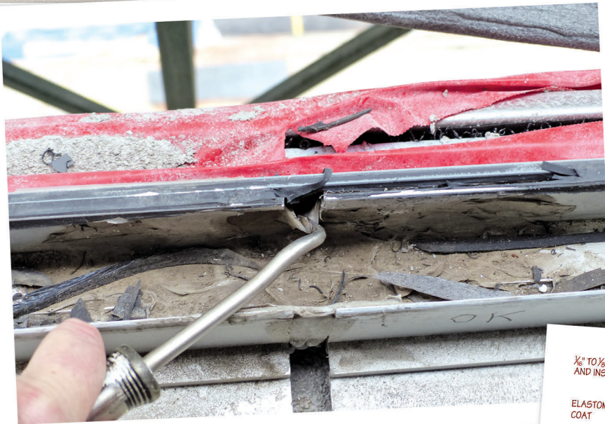
Figure 5 – Failure of retrofitted sealant at splices.
