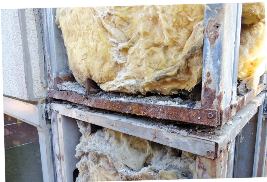
Figure 21 – Corroded light-gauge steel-framing members.
